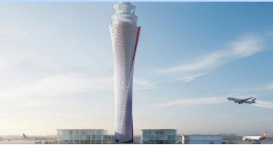
GIA BINH AIRPORT PROGRESS
