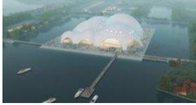
OPERA HOUSE PROGRESS
