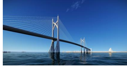
CAN GIO BRIDGE PROGRESS
