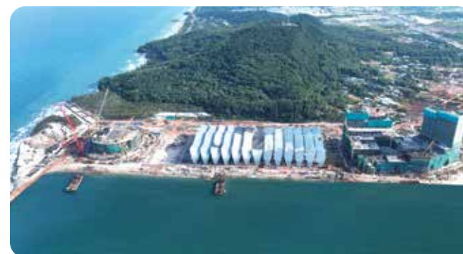
Panoramic View of the Phu Quoc Coastal Megasite: Simultaneous Construction Across Sub-Zones S2, S3, and the S4 Tower
