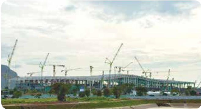
Panoramic View of the Terminal 2 Construction Site
