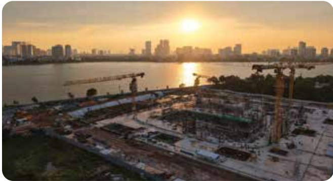
Panoramic View of the Construction Site Executing Complex Orchestra Pit and Foundation Structures Under the West Lake Sunset
