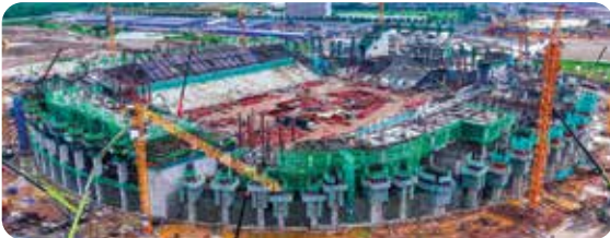
Accelerated 270-Day Construction Progress: Rapid Installation of 84 Perimeter Columns and 9-Tier FIFA-Standard Grandstand Structures
