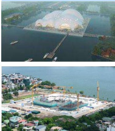
OPERA HOUSE PROGRESS
