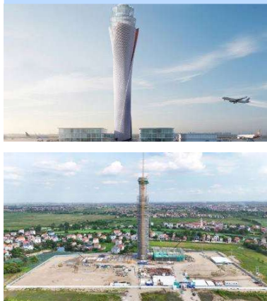
GIA BINH AIRPORT PROGRESS
