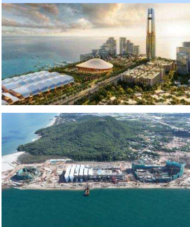
APEC PHU QUOC PROGRESS
