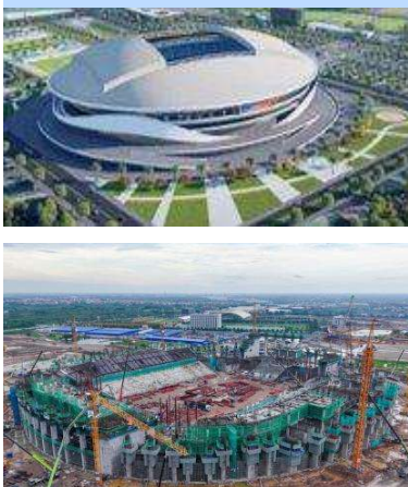
PVF STADIUM PROGRESS
