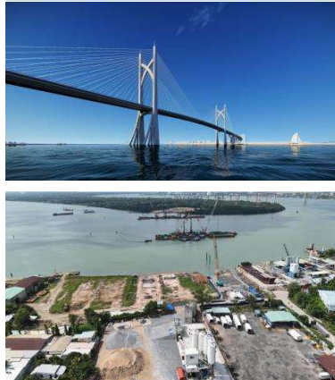
CAN GIO BRIDGE PROGRESS
