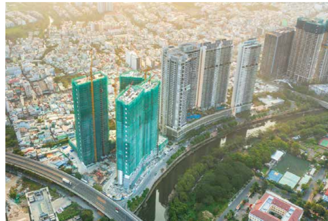
The Infiniti (Riviera Point – Phase 1C) in Ho Chi Minh City is Vietnam's first high-rise project to use CO 2 -mineralized concrete, helping reduce carbon emissions during construction.
