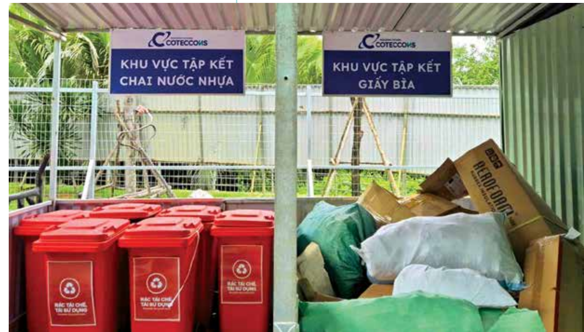
Waste collection and segregation area at a Coteccons construction site, supporting effective waste management at source.
