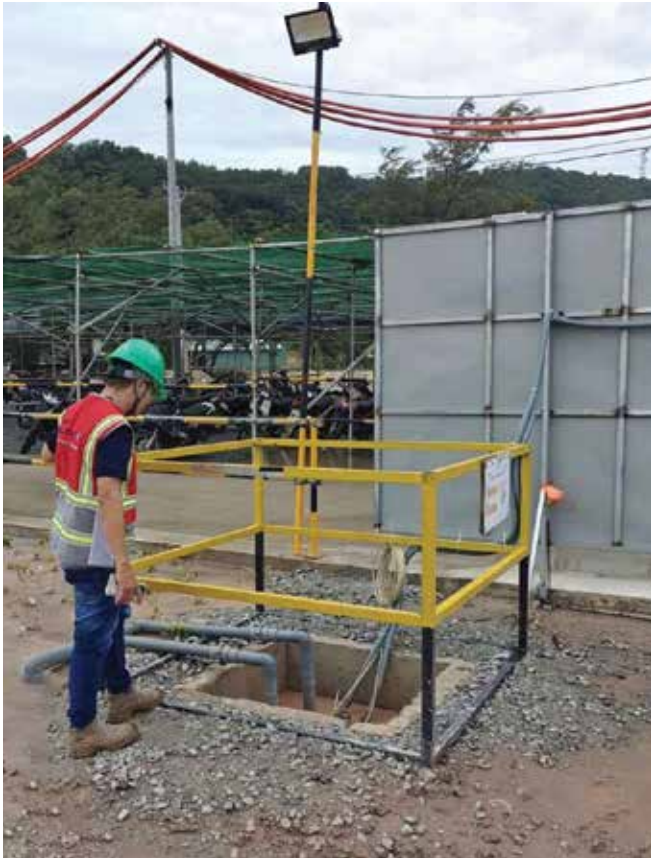
Environmental monitoring and inspection of the wastewater collection and treatment system at the APEC Convention Center project in An Giang.
