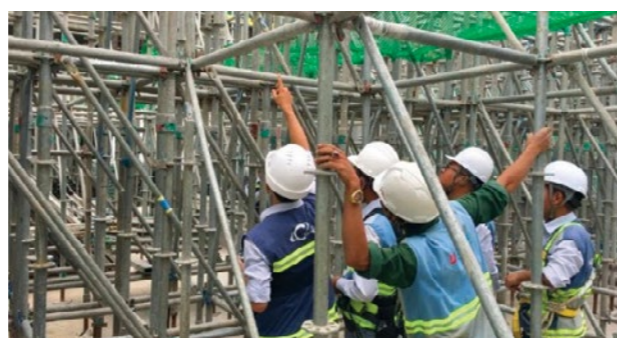
Conduct acceptance test of special components
