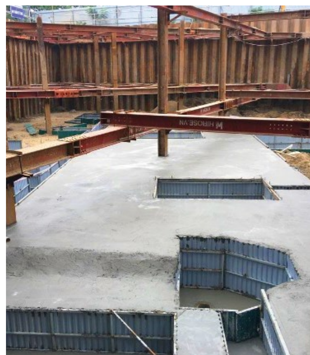
Install tole formwork for the basement foundation
