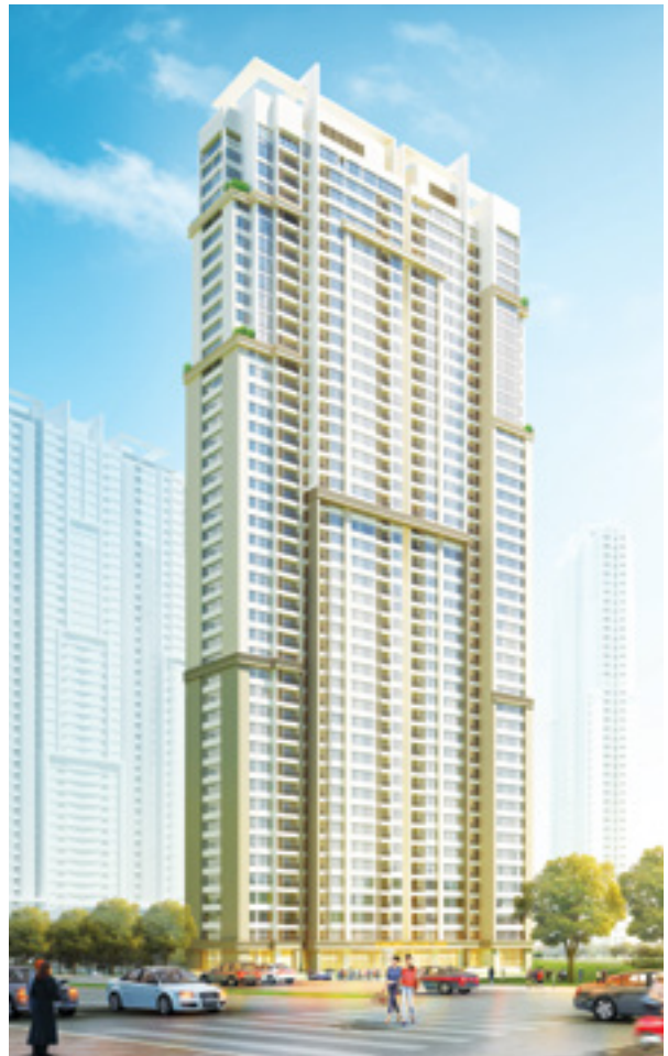
Vinhomes Central Park - TP.HCM
