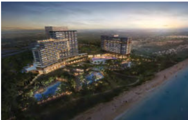
Won the bid and commenced construction for the VND 7,000 billion Casino at the South of Hoi An
