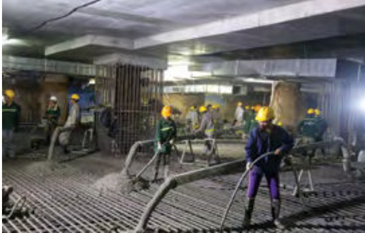
32,305m 3 concrete and 45.5 hours - The Biggest Concrete Construction at Coteccons
