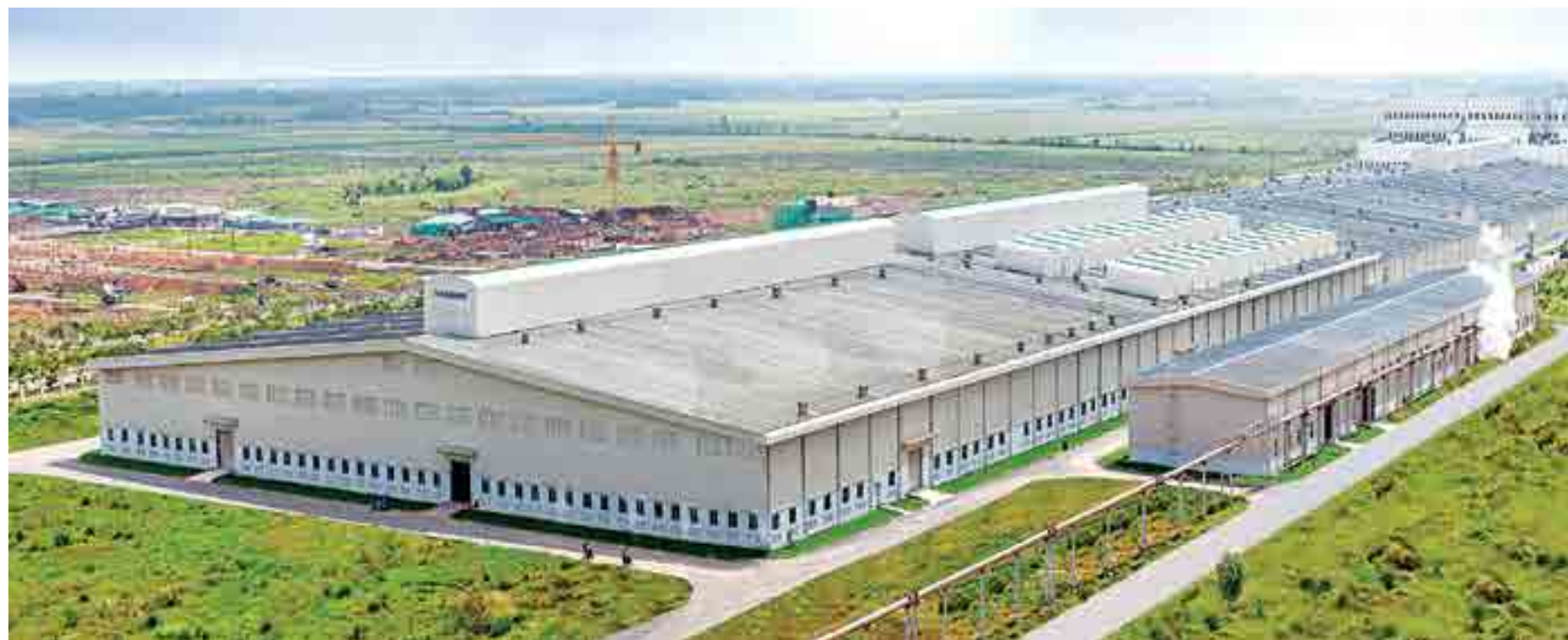
Salun Factory at Phuoc Dong Industrial Park - Tay Ninh
