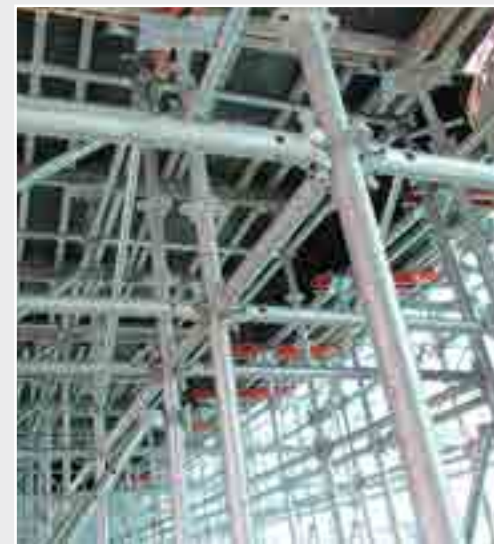
Ringlock scaffolding system research and application
