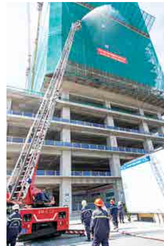
On-site fire drill
