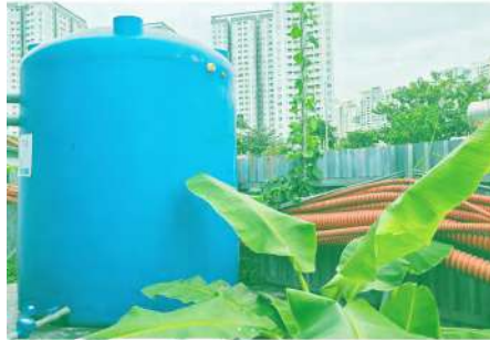
Rainwater collection tank for sanitation and watering plants
