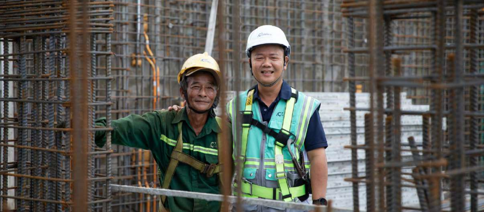
Coteccons' investment in OHS (occupational health and safety) at the Suntory PepsiCo project amounts to approximately 0.2% of the total project value.
