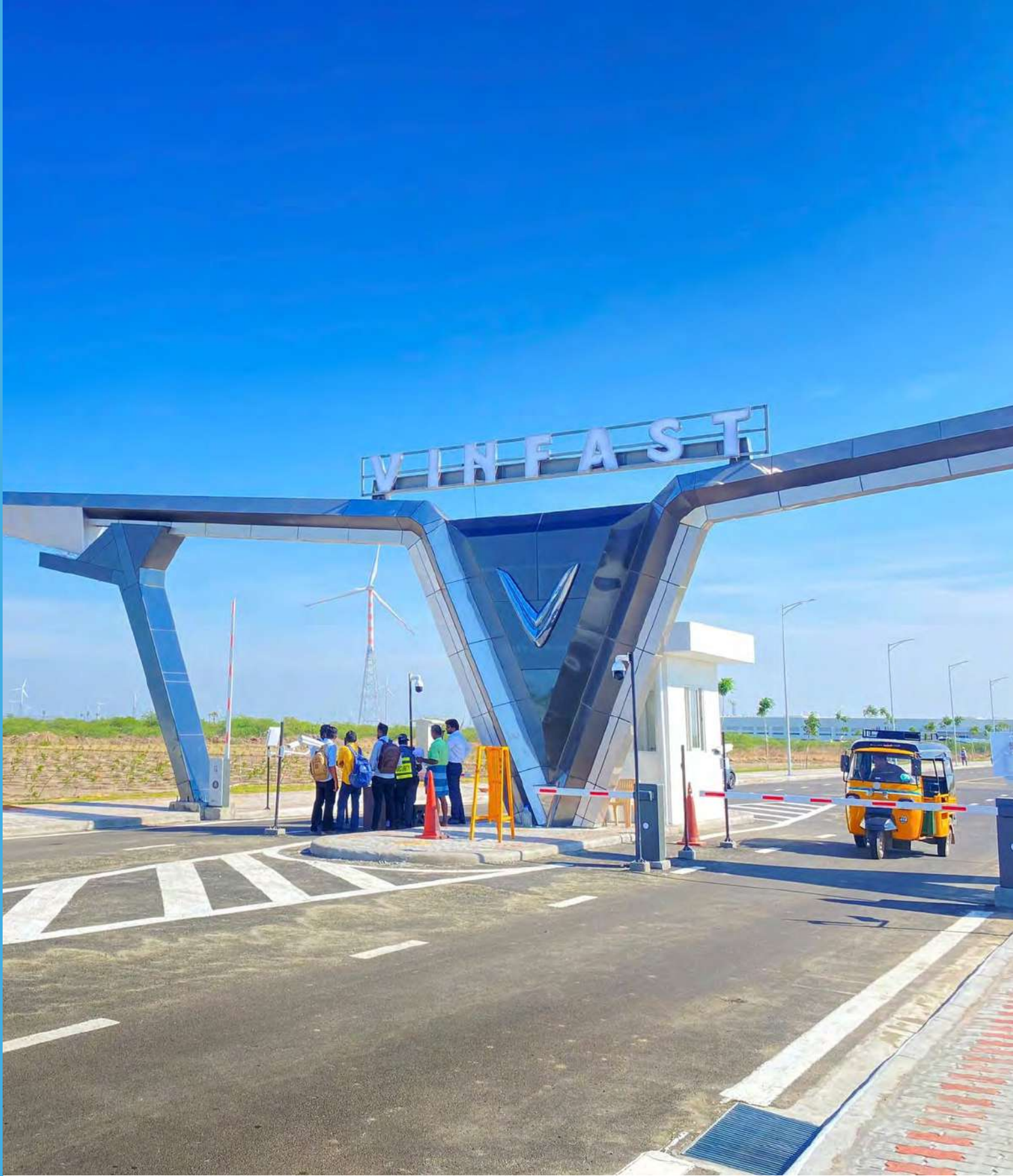
VinFast factory project in India
